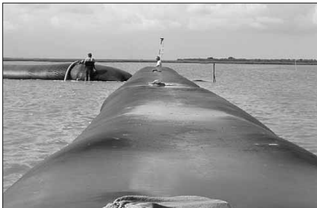
Geo-textile tube being filled by hydraulic dredge.
