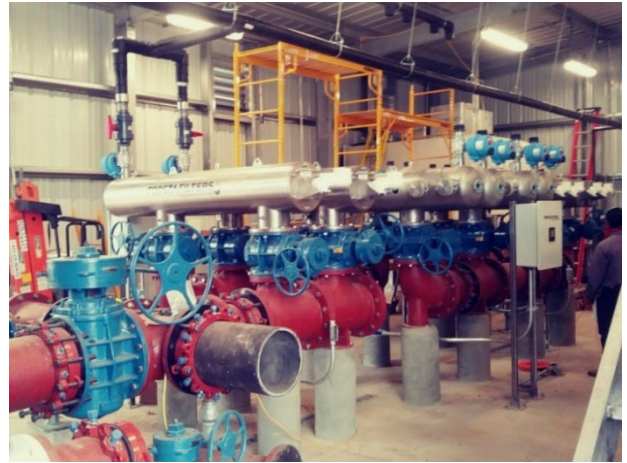
Micro-filtration system constructed at the Possum Kingdom Fish Hatchery.
