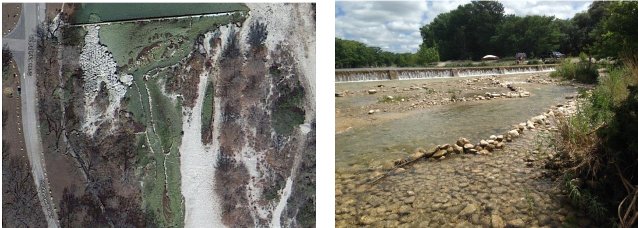
Figure 7. Aerial imagery from 2012 (left photograph) shows the Frio River below the dam at Garner State Park with extensive man-made rock walls diverting flow within the streambed. The right image was taken in June 2014, less than two weeks after an 8,000 cfs flood pulse moved through the system. The rock walls remained largely intact after this flood event.
