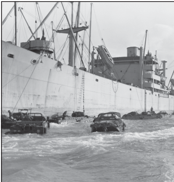
Figure 20. Army "ducks" which operate from ship to shore carrying cargo from Liberty Ships to shore are shown being loaded with gasoline drums, Bassin Darse Nord, Le Havre, France, 470th and 819th Amph. Truck Co., Nov. 15, 1944 (National Archives).
