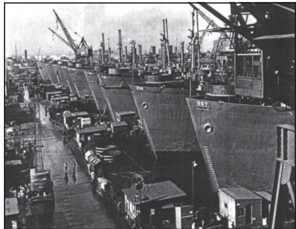
Figure 2. Liberty Ship production line at the California Shipbuilding Corp. Courtesy of the Library of Congress (Hoehling 1990).
