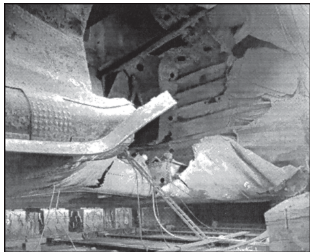
Figure 32. Damage to the John Worthington's hull at Tank No. 8. The explosion punctured the bulkheads fore and aft of Tank 8, flooding Tanks 7 and 9 as well. Photo probably taken after her arrival in Texas on June 21, 1943. (From Standard Oil of New Jersey, The Esso Fleet in World War II .)
