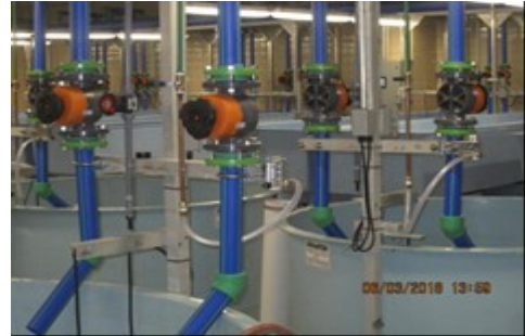
A newly renovated incubation system will improve operations at A.E. Wood Hatchery.
