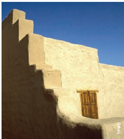
Fort Leaton State Historic Site
