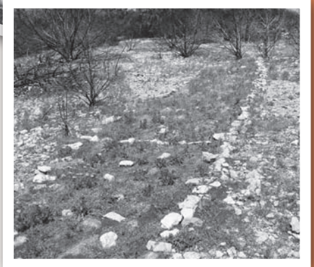
Straw erosion and seed mats were laid. After six months, results are evident.
