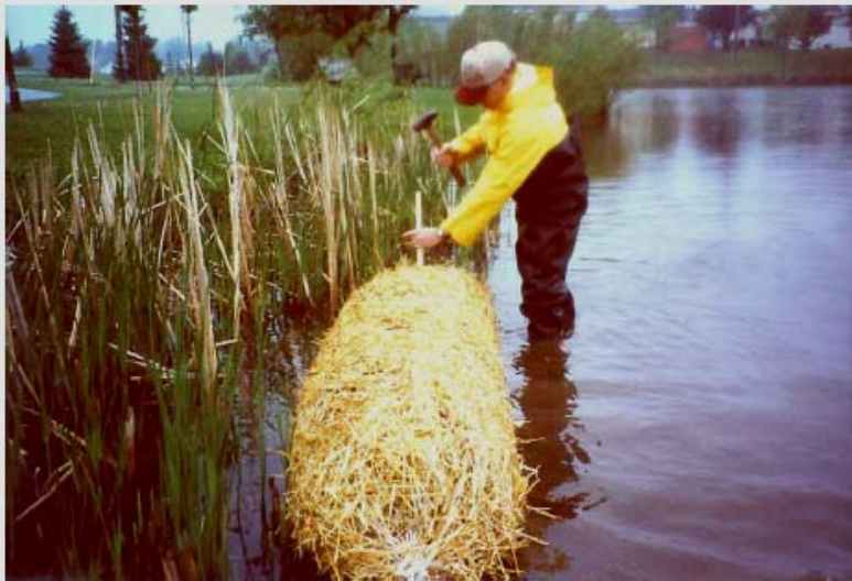
Figure 2. A large barley bag being anchored into a lake. Photo courtesy of Steve McComas, Blue Water Science, St. Paul, MN.
