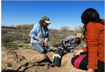
Burrow entrances must lay level and perpendicular to the ground preventing rain from entering the burrows. Secure the entrance with rocks to control erosion and deter digging mammals.
