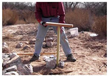
Construct a shade structure from a 2X2' piece of plywood and 4' sections of rebar and place close to or over the burrow entrance. Paint both sides of the shade structure prior to installation to protect the wood. Caulk the rebar to the wooden shade structure in the field.
